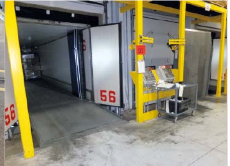
Vertical-storing leveler allows loading dock doors to close on the pit floor.
