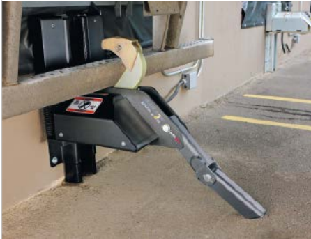
A vehicle restraint wraps around a trailer's RIG, securing the trailer to the loading dock.
