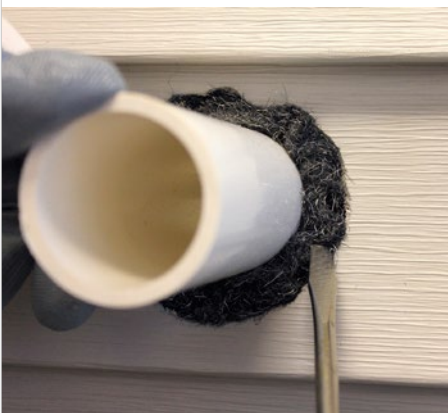
Specialized, rodent-proof products, like Xcluder fill fabric, are fundamental to proper exclusion.
