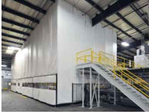
Humidity walls separate higher and lower humidity spaces.
