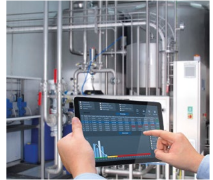
The Diversey CIPTEC can provide users with precise CIP monitoring to allow for shortened CIP cycles.
