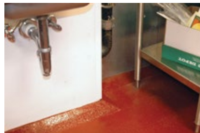
Repair specifications may include recommendations for incorporating cove bases (shown), which can provide seamless transitions from floors to walls, to eliminate a common bacteria harborage point.
