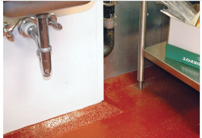
Figure 2. A cant base creates a seamless transition from walls to floors to promote drainage and eliminate the typical 90-degree transition where bacteria can become trapped.
