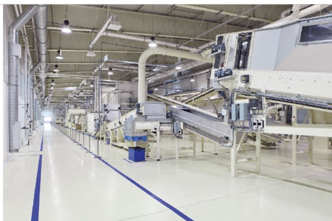
Fig 3. Metal ceilings, railings, columns, and other steel surfaces in food processing and storage areas should be coated and maintained to prevent rust and paint chips from breaking loose and contaminating products.
